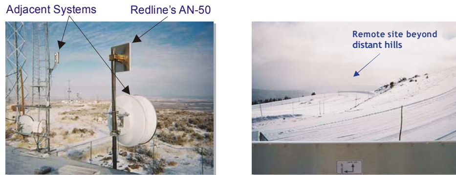
Figure 5 Long range deployment co-existing with co-located in-band systems.
